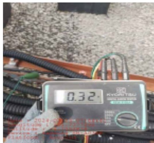
IGB / INDOOR SHELTER
